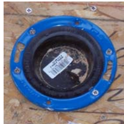
Closet Ring screwed into Toilet Anchor
