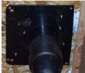
Trimmed Toilet Anchor
